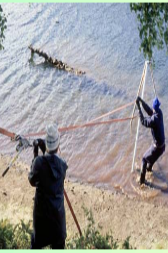
Winches and a rigid tripod were used for pulling up the logs.
